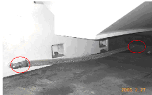
Connect two water pipes link between base and coolant tank
