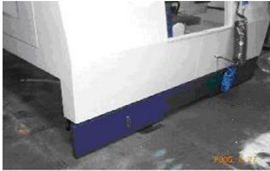
After leveling machine and fit coolant tank and chih conveyor
